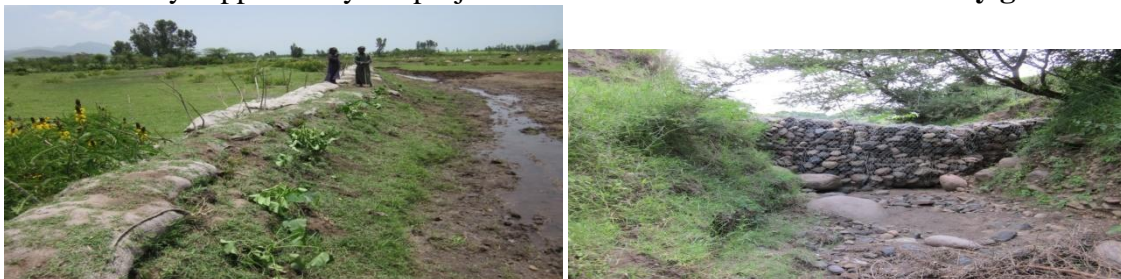
Felana river flood control by sacks & vetiver grass in kebele 31 &32
